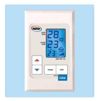
The controller screen will return to the main operating screen (shown here on left). The system may alarm again if it can still sense smoke. You will need to repeat the steps above to reset the system to the main screen.
